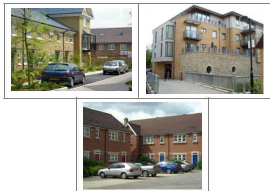
From top left: (1) Off-plot parking, Reliance Way, Oxford; (2) Basement parking, Woodin's Way, Oxford (3) Forecourt parking, Waterside, Oxford
